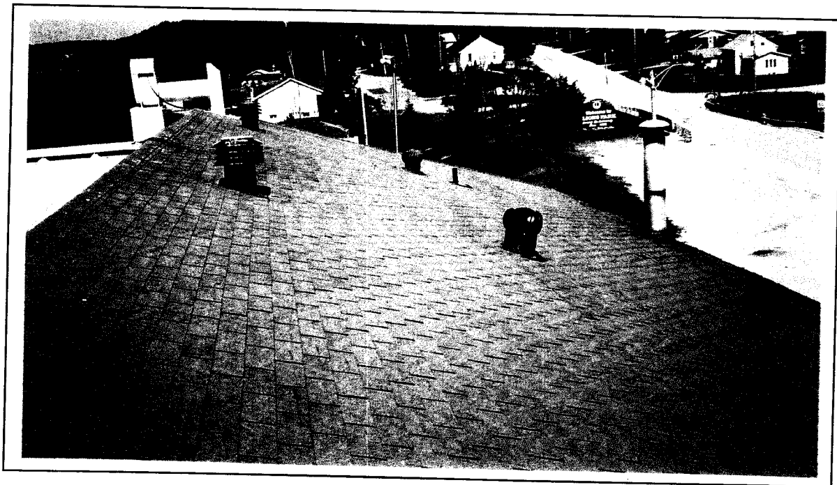
VIEW OF ROOF
